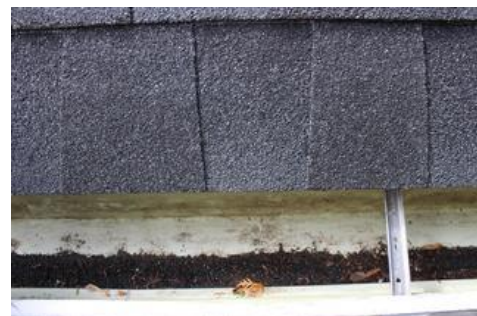
Newly installed shingles
