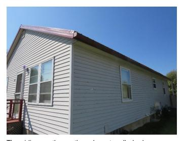
The siding on the north and west walls had numerous fractures. The siding on the north and west walls will need to be removed and replaced.
