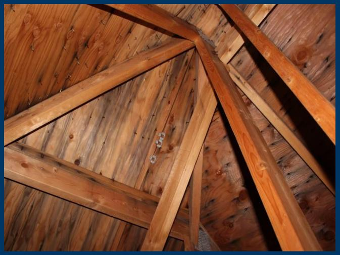
Origin (Source + Path) = Indoor Humidity + through the ceiling + condensing on cold roof
