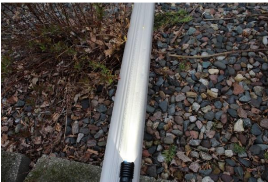
Horizontal Extensions of Downspouts
