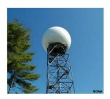
The image below is of a radar within the protective dome. The radar is a two part system that sends out a signal and reads the returning signal.
