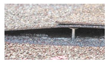
The nail actually pops up and out of the wood deck causing the shingle to be lifted. The nail backs out of the wood deck where it once had been adequately inserted to the correct depth.
