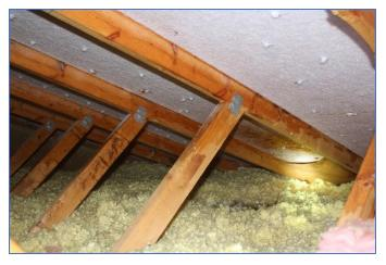
Frost can build up in the attic uniformly and more concentrated at air leaks. When the temperature rises above 32 degrees at the frost location, that frost melts and it can appear as a leak. The water rushes out and then stops. This "leak" can be excessive when the temperatures dramatically change, as is common during the warming up a cold house where the temperature has been substantially reduced when owners where not home for extended periods of time.
